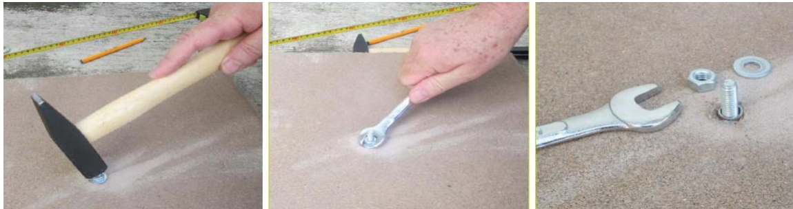
Figura # 24: Táquete en el orificio https://imgv2-2-f.scribdassets.com/img/document/228339361/original/
