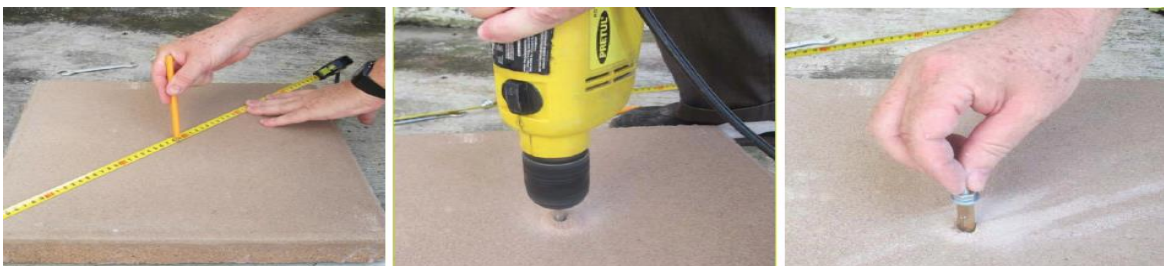
Figura # 23: Táquete en el orificio https://imgv2-2-f.scribdassets.com/img/document/228339361/original/
