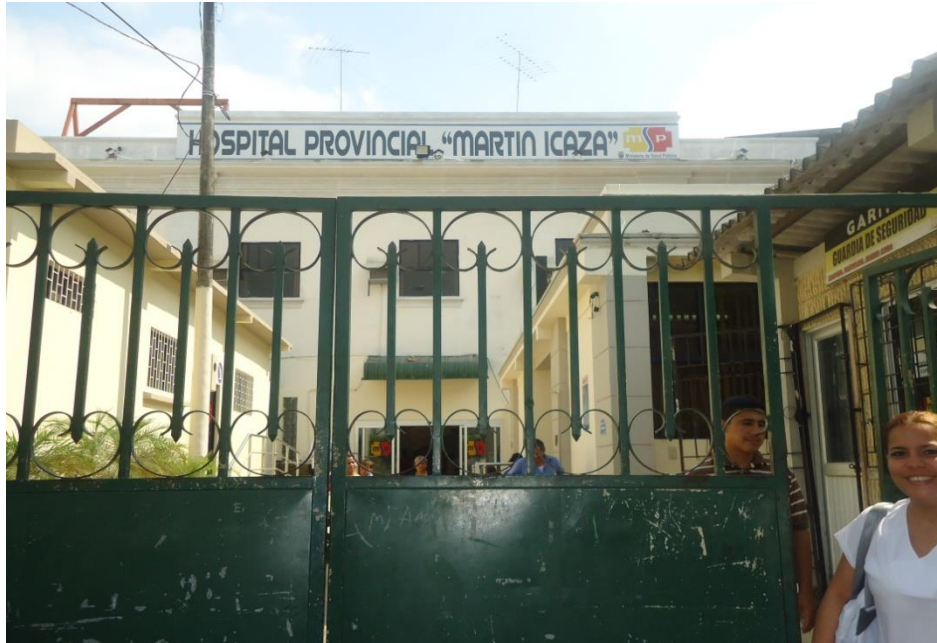
ENTRADA HOSPITAL MARTIN ICAZA
